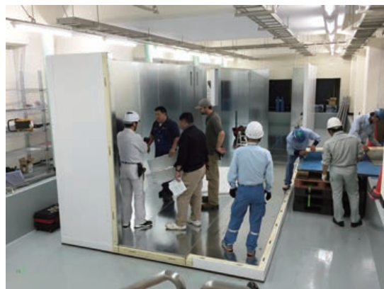
Workers erect framework for new robotic biorepository
