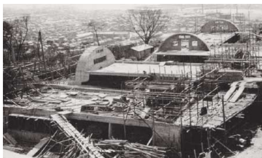
1949 Construction in progress at Hijiyama
